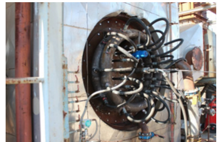
Burner installed on a steam generator
